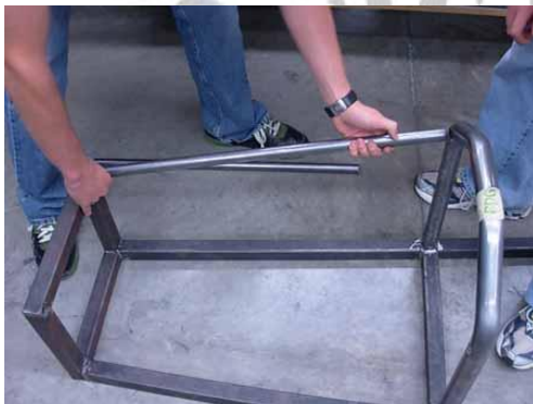
Fitting in one of the side supports on the chassis
